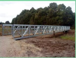
Another recently completed project supplied and installed by GRDC is this 32 x 2.0m Steel Truss Footbridge located a the Sale Common in South East Victoria. The old derelict footbridge was demolished and removed from the area making way for the new footbridge. Comprising of hot dipped galvanised steel trusses, bearers and joists with Banksia panel and treated pine joists and decking the new footbridge is practical and eye catching.
