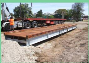
This 10x1.5m steel I-Beam footbridge was recently installed at Possy Newland near Little River. Fabricated entirely in our Port Melbourne factory this bridge was transported to site and craned onto concrete abutments. Featuring hot dipped galvanised bearers, LOSP treated pine joists and hardwood decking, this cute little bridge would be ideal for your next space project!
