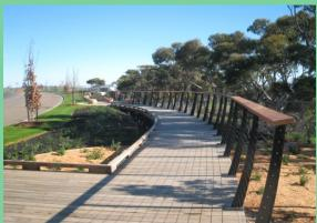
In Geelong, GR Design & Construct recently constructed this boardwalk for a local developer which consisted of hardwood bearers and joists, timber caprail and all stainless steel fixings. Once the boardwalk was completed we retrofitted the powdercoated, stainless steel handrail with a timber caprail for safety reasons. Another GR Design & Construct project completed on time and within budget.
