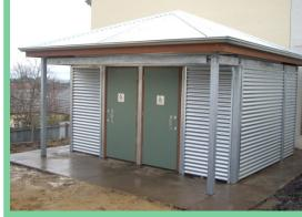
This Twin Disabled Restroom was designed and constructed for the Daylesford Neighbourhood Centre. The pyramid roof, hot dipped galvanised posts and Zincalume external cladding were chosen to match the surrounding buildings. The internal cladding was white painted plywood to give it a modern, clean look.
