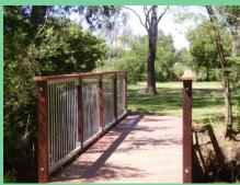
GRDC used local contractors to install this 10 x 2m Steel I-Beam Footbridge at the refurbished Port of Maffra. The footbridge featured a timber & steel handrail and hardwood decking.
