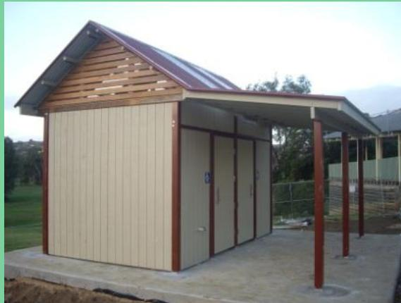
GRDC designed this 2D restroom with service duct to fit in with the surrounding infrastructure. External cladding, painted shadow clad, internal painted fibre cement sheeting and manor red steel posts.
