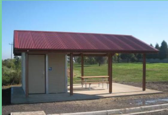
This Custom Shroom (Shelter / Restroom) was designed and constructed in conjunction with local Council. Comprising of a ID Restroom facility with service duct, all stainless hardware, pans and cisterns, this shroom was connected to mains sewage. There is also ample room for picnic tables and seating which are protected from the elements. Ideal for walking trails, remote bus stops and recreation reserves.
