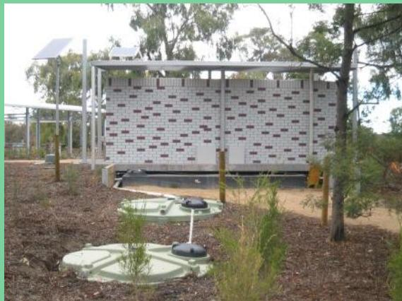
Royal Botanic Gardens, Cranbourne required a large restroom facility but there was no mains sewer available to connect to. This custom hybrid alternate waste system was the perfect solution with one large primary tank (under the suspended slab) a secondary tank and one holding tank. The hybrid system is a water based treatment facility ideal for remote and environmentally sensitive locations and maintenance free.
