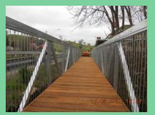
This is a classic example of GRDC's ability to fabricate products in our Port Melbourne factory therefore reducing on site works and environment al impact. The bridge was fully assembled prior to being picked up, delivered and dropped onto concrete abutments by a crane truck for low cost supply and installation.
